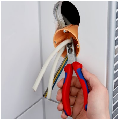
Stripping deep down in a flush-mounted junction box
